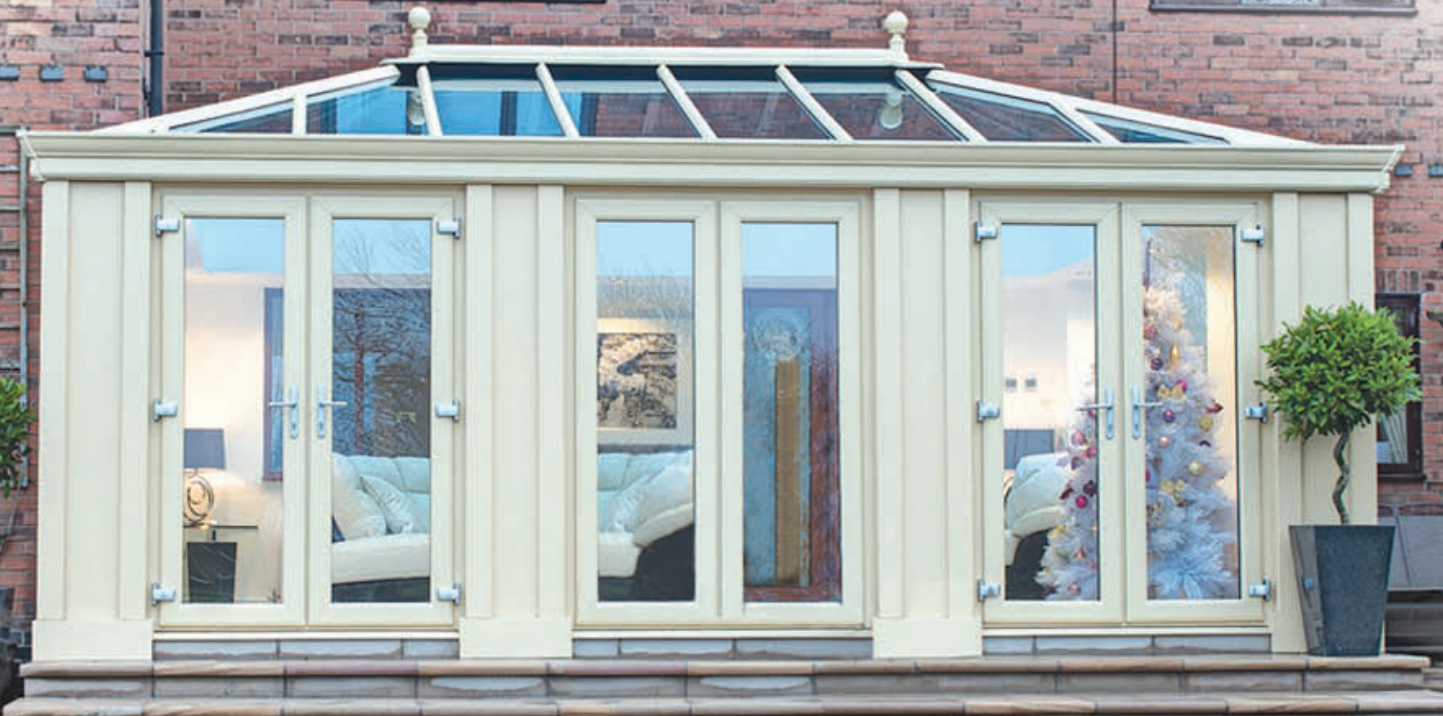
Mottram plus Loggia Glazed Extension
